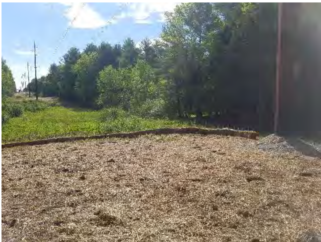
Fig 2: Str. 65 work area restored. Viewing east. (05-28-20).
