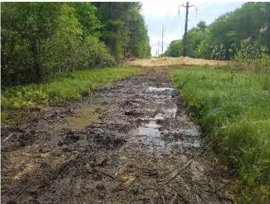
Fig 18: Timber mats removed from access road to Str. 75, through wetland DW21 Viewing east. (06-03-20).
