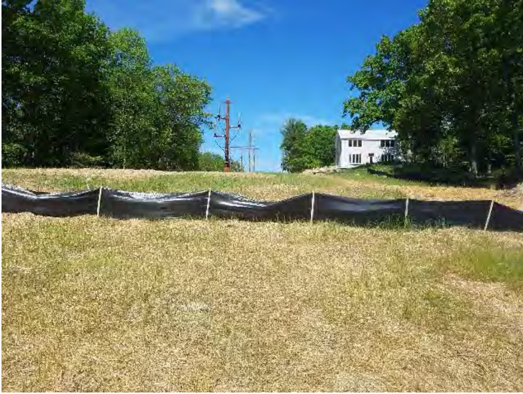
Fig 13: Vegetation on slope at Getchell property/west side of the Bay. Viewing west. (06-02-20).
