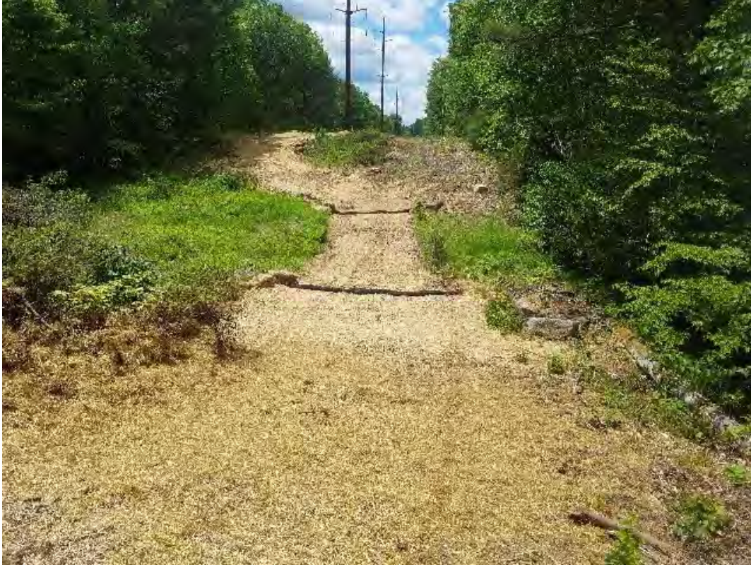
Fig 11: Restored access road between Strs. 65-66 and through wetland DW9. Viewing west. (06-01-20).
