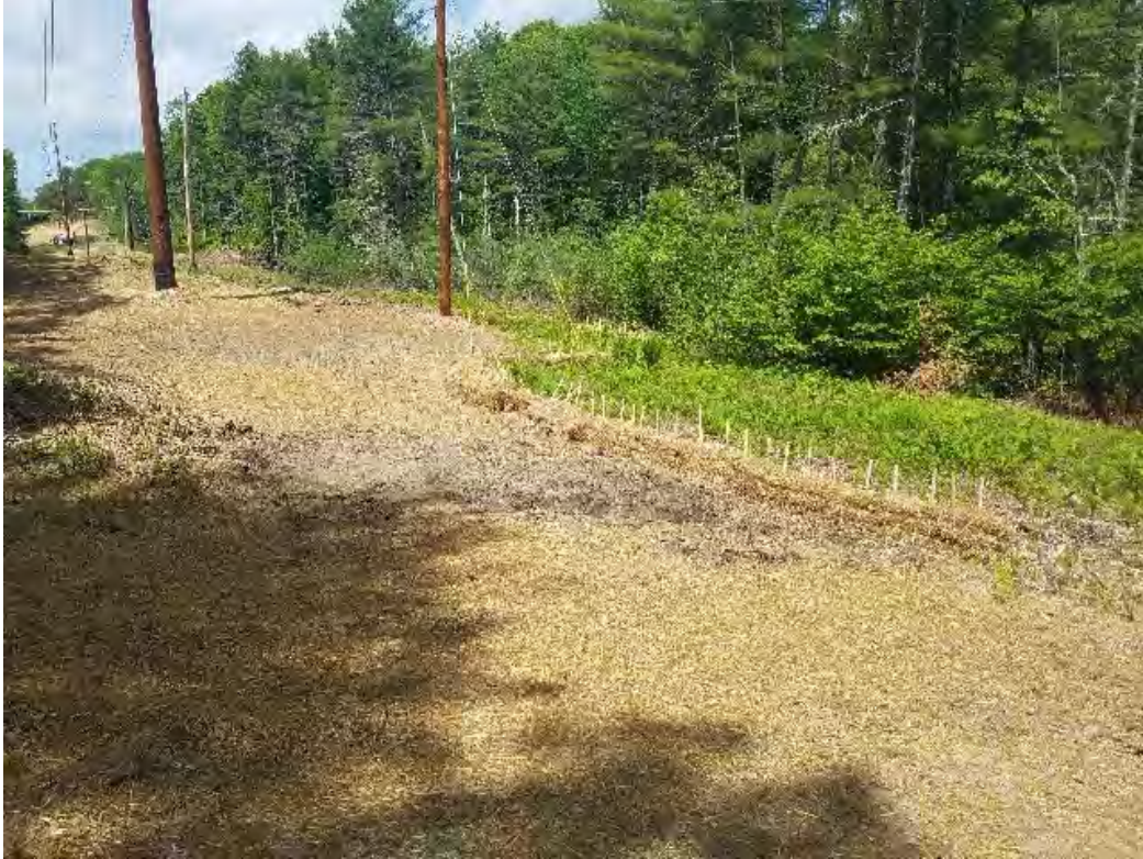
Fig 7: Str. 62 work area restored. Viewing west. (05-29-20).
