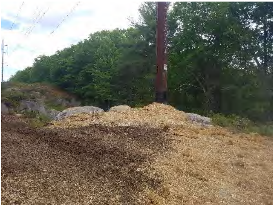
Fig 12: Str. 79 work area restored. Viewing east. (06-01-20).
