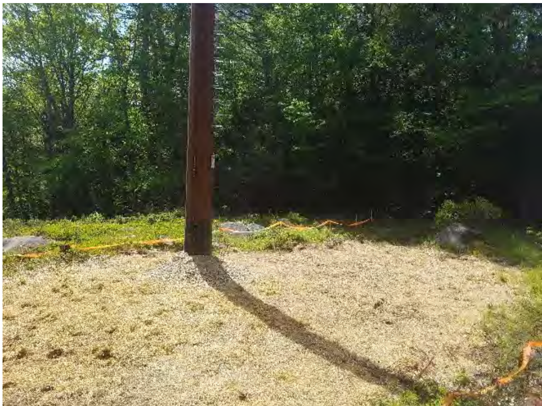
Fig 4: Str. 81 work area restored. Viewing south. (05-28-20).
