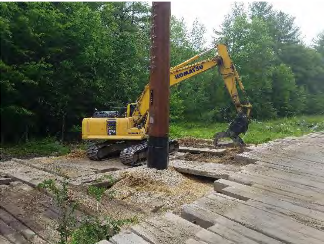
Fig 16: Removing timber mats used for work pad at Str. 89. Viewing northeast. (06-03-20).
