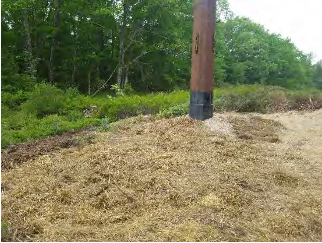
Fig 5: Str. 81 work area restored. Viewing southwest. (05-29-20).
