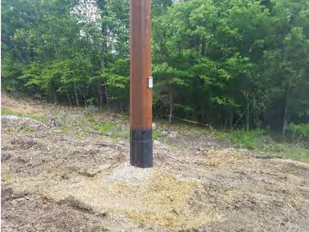
Fig 17: Timber mats removed around Str. 89. Viewing northeast. (06-03-20).
