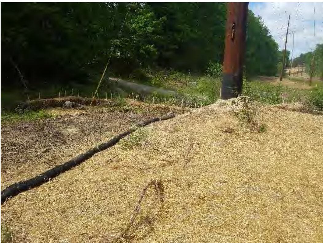
Fig 6: Str. 63 work area restored. Viewing west. (05-29-20).
