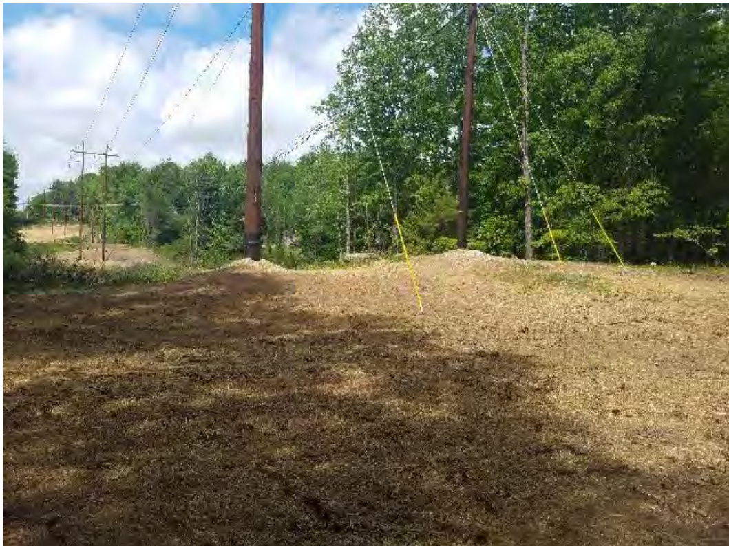
Fig 8: Str. 61 work area restored. Viewing west. (05-29-20).
